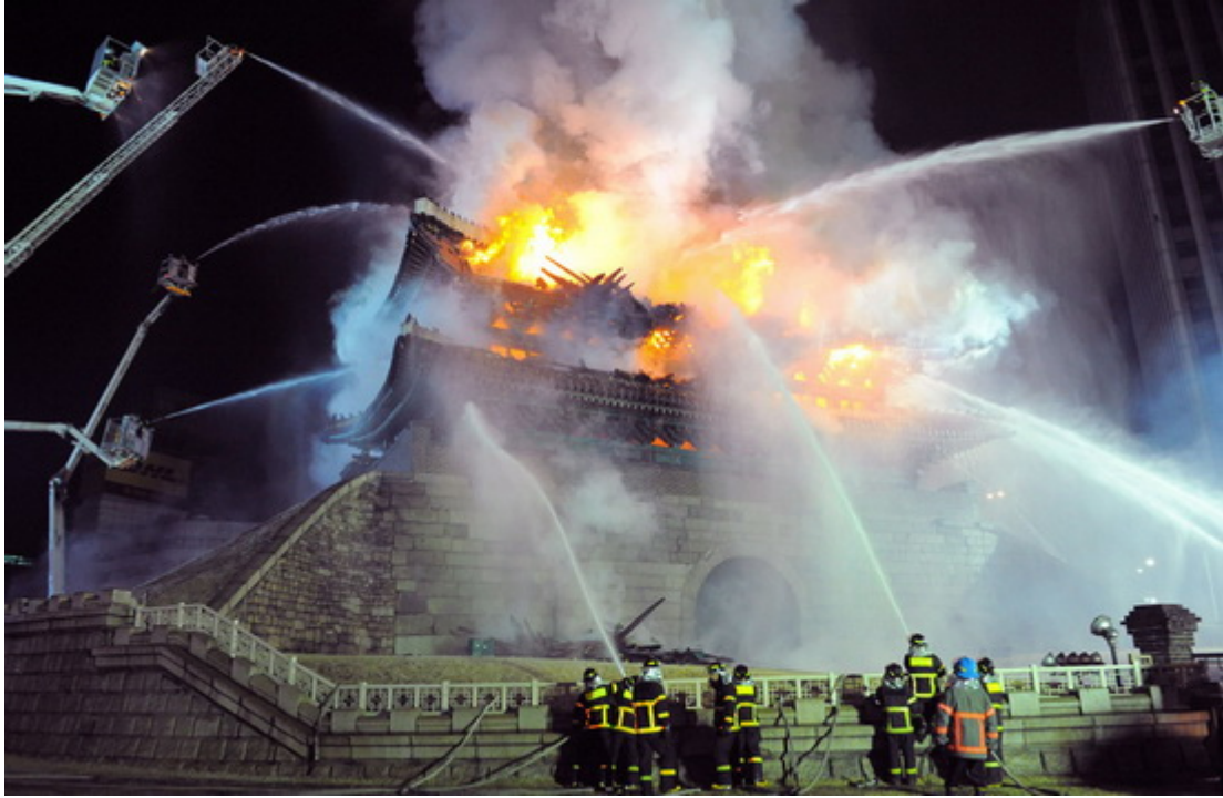
9. Firefighters battle a blaze at the Namdaemun gate, one of South Korea's most historic sites, in central Seoul, on February 11, 2008. An arsonist started the fire, destroying the gate - the oldest wooden structure in Seoul, first constructed in 1398 and rebuilt in 1447. (Kim Jae-hwan/AFP/Getty Images)
